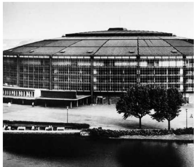
The roof of the Westfalenhalle in Dortmund, which was built in 1952, exemplifies how untreated aluminium surfaces can withstand the elements without any difficulty. (Fig. 1)
